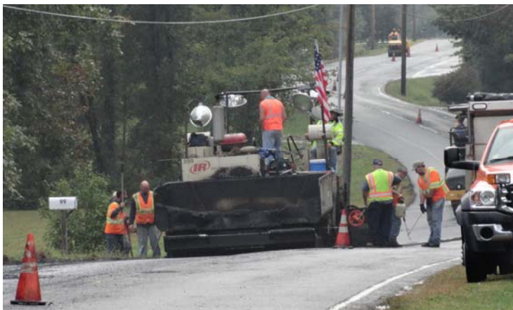
Paving Operation on CR 637
