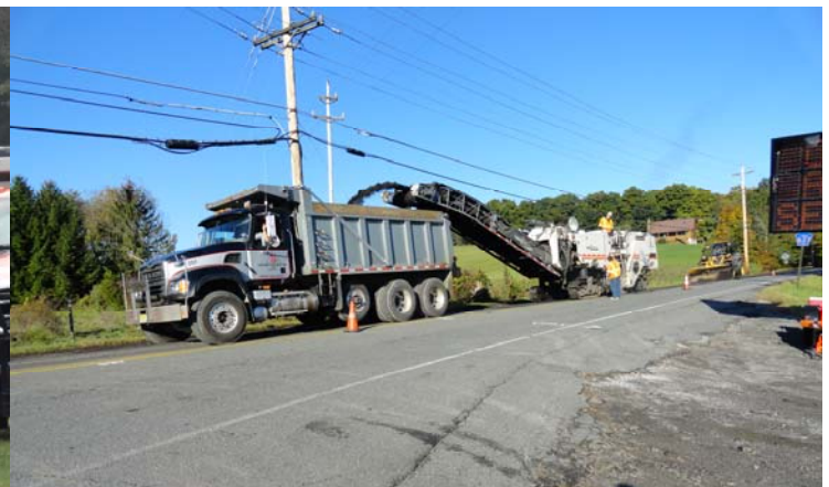
Milling Operation on CR 637
